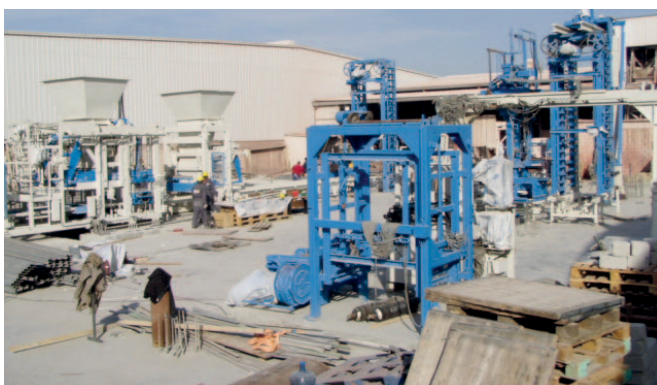
Mechanical erection of the Schlosser SV 30 blockmaking plant
