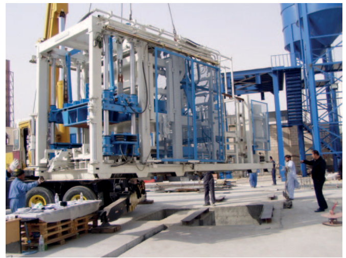
Putting of the Schlosser SV 30 block making machine on the prepared foundation
