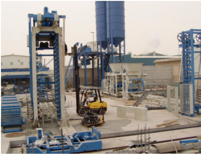
Once Bonyan finished the foundations, Contec started the mechanical installation.
