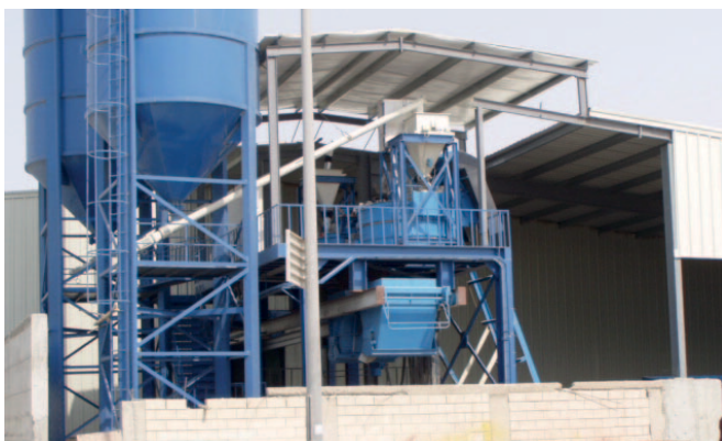
The double feeding bucket conveyor transports concrete from the two OMG/Sicoma concrete mixers to the block making machine.
